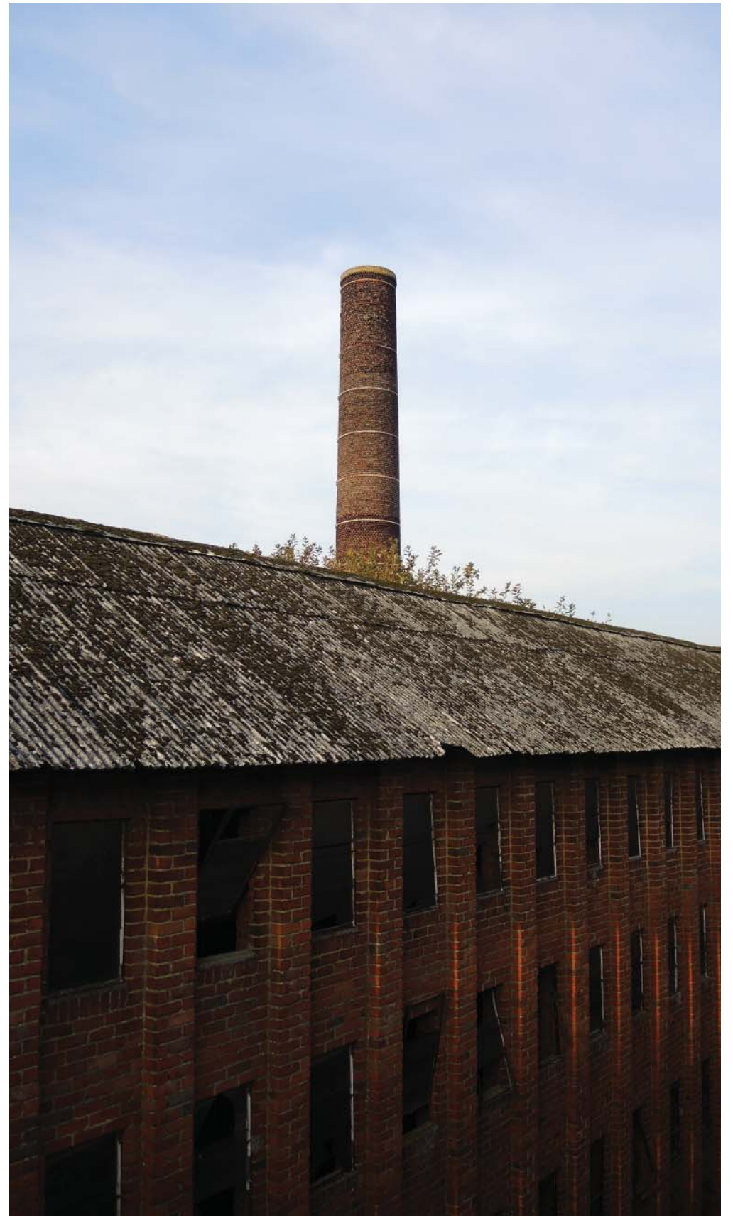
Chimney seen from between drying sheds - Artit Markshom ©
