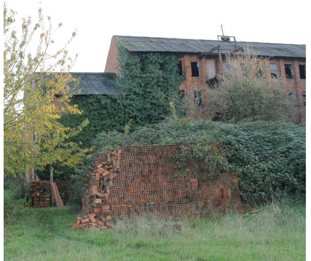
Vining plants on north end of drying shed
