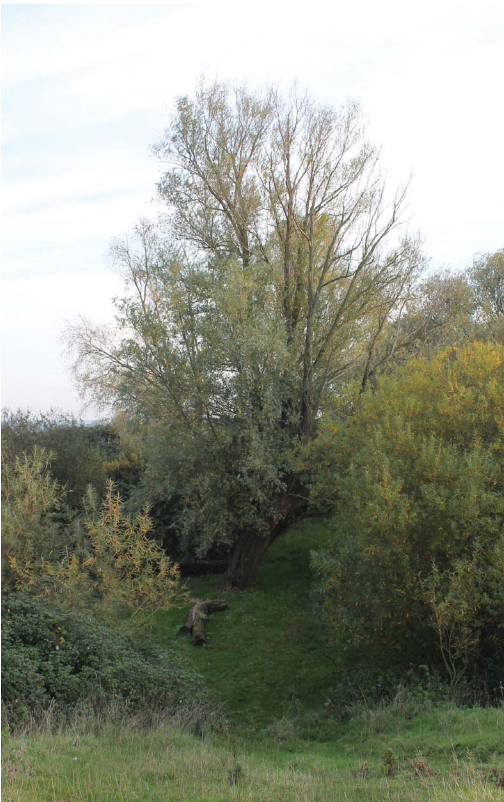
View of tree clearing at bottom of claypit
